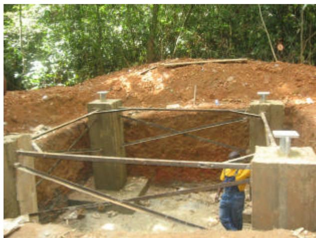
Figure 1: Basement for the new tower for monitoring CO<sub>2</sub> fluxes in Ghana.
